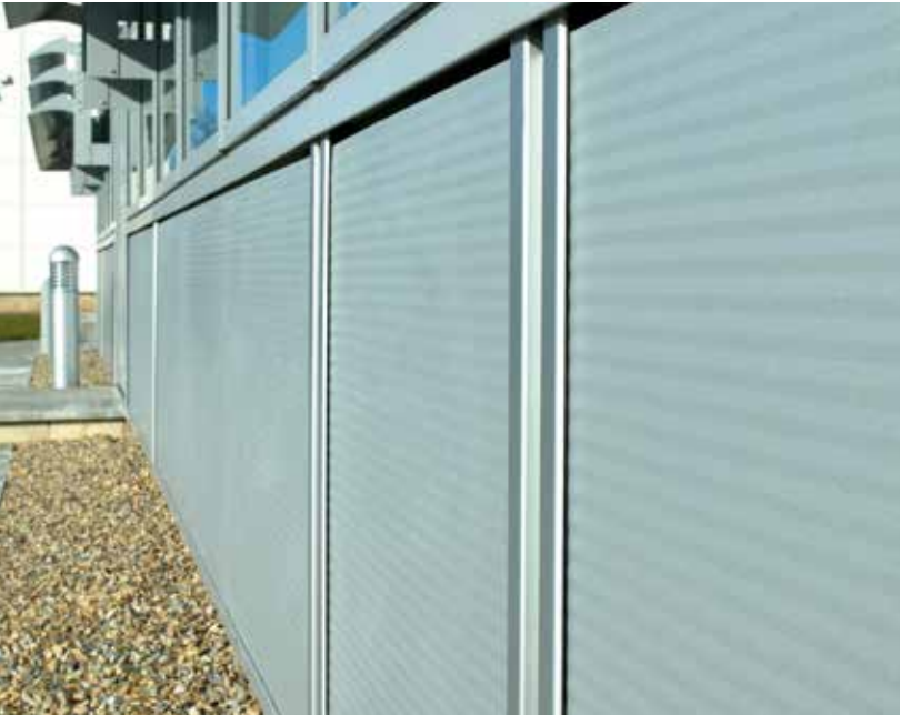
Sill extrusion
